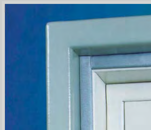
Fire Seal around Door
